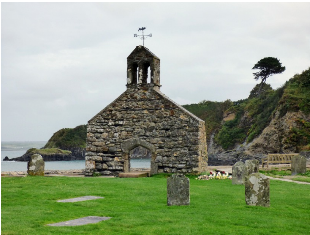
Cwm yr Eglwys — gable end, some of the churchyard, and some of the graves remain in position after a stormy past
